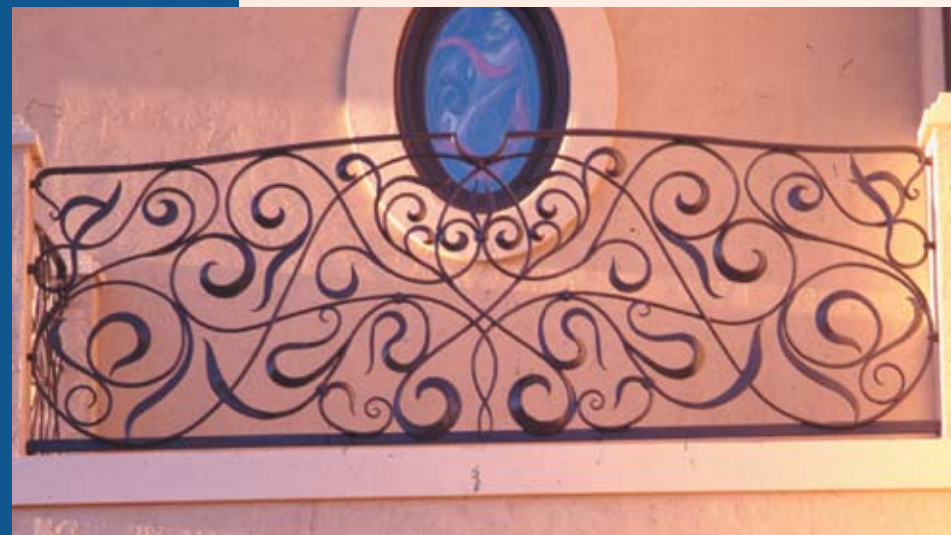
Walt Hull, Walt Hull Iron Work, Lawrence, Kansas Balcony railing in mild steel. 8'6" l x 3'h. Designed by Walt Hull and executed by Kate Dinneen. Photos by Walt Hull.
