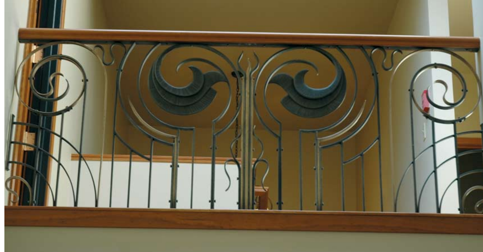
Iron and bronze balcony railing in a lawyer's office. The handrail is cherry.
