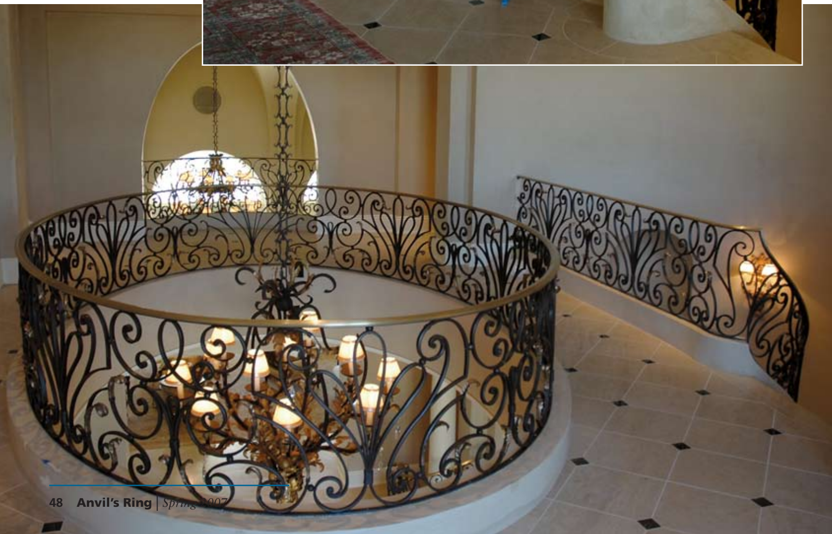
Railing on the second floor with a large oval opening to the lobby.
