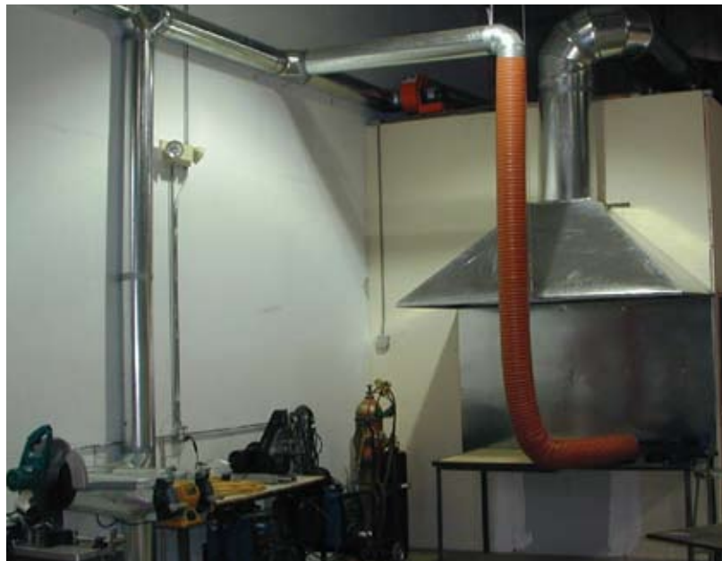
The grinding and welding area is well equipped with a ventilation system.
