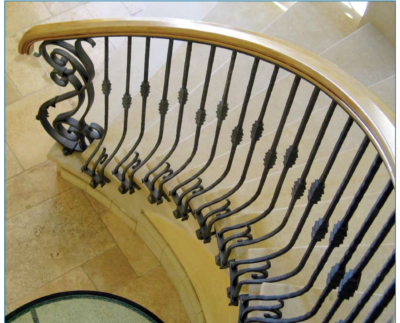
Interior curved railing terminals and forged balusters. A lateral mount was used to avoid dealing with stone steps.
