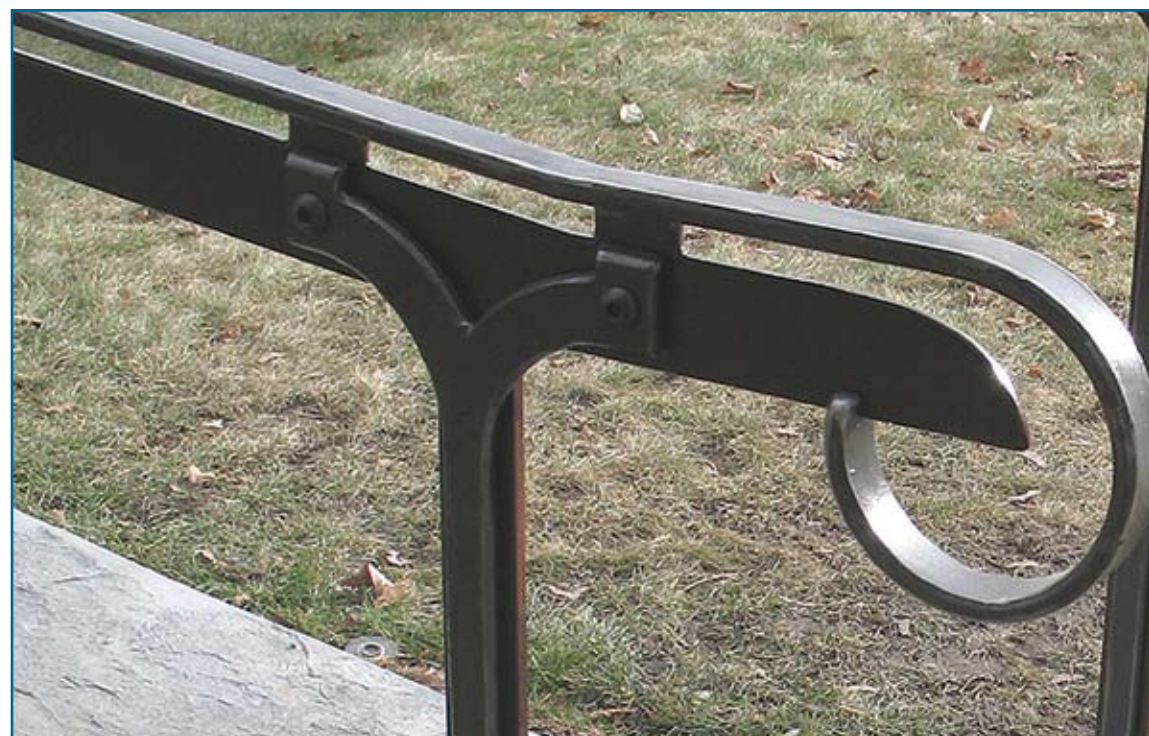
Exterior entry railing detail.
