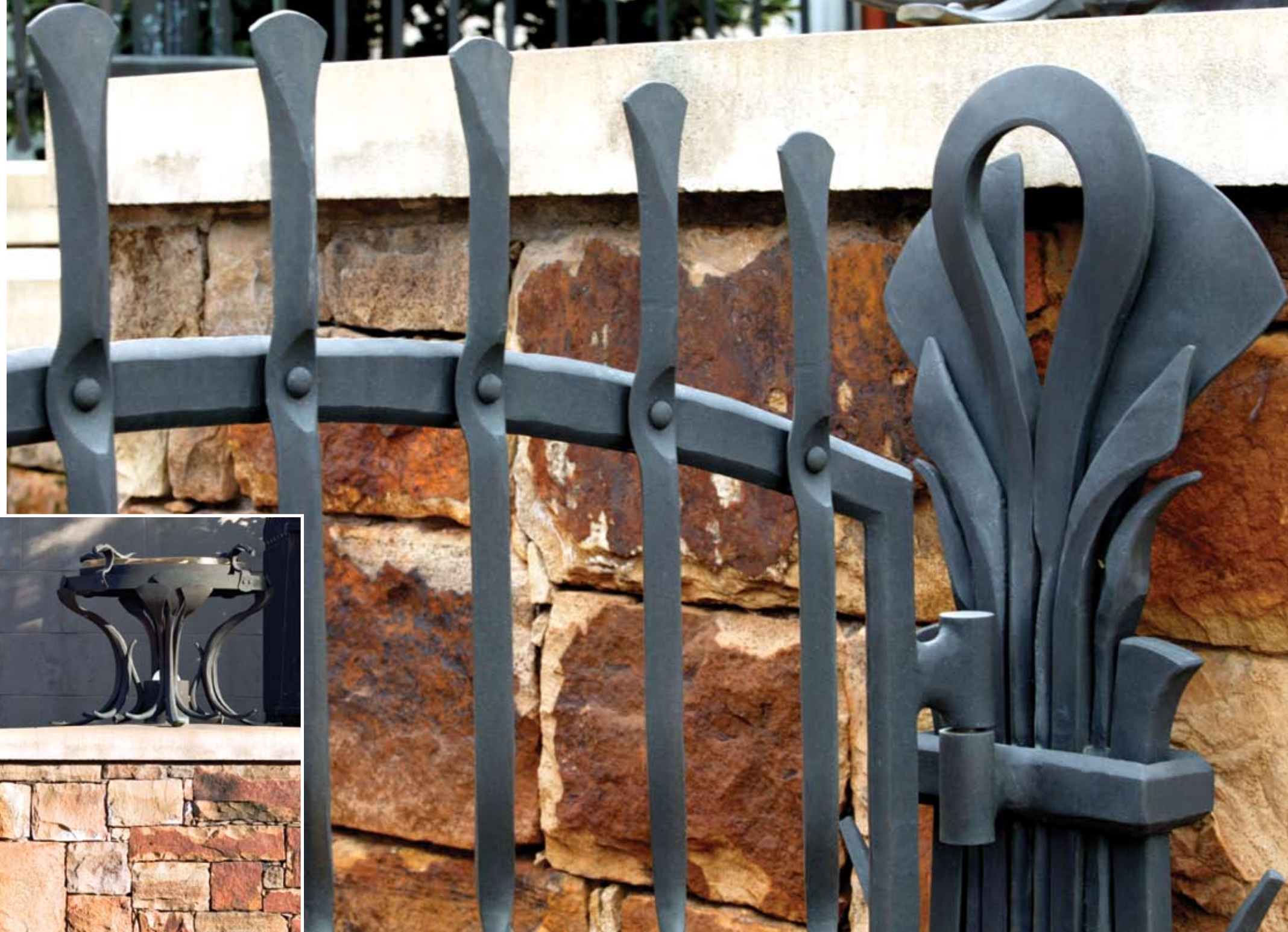
Silicon bronze (alloy 665) detail of gate post and forged framework of gate. Frame is forged from 1x1 sq. bar to a hex shape. Balusters are 3/4 sq. with fullered dimple and riveted connection.
