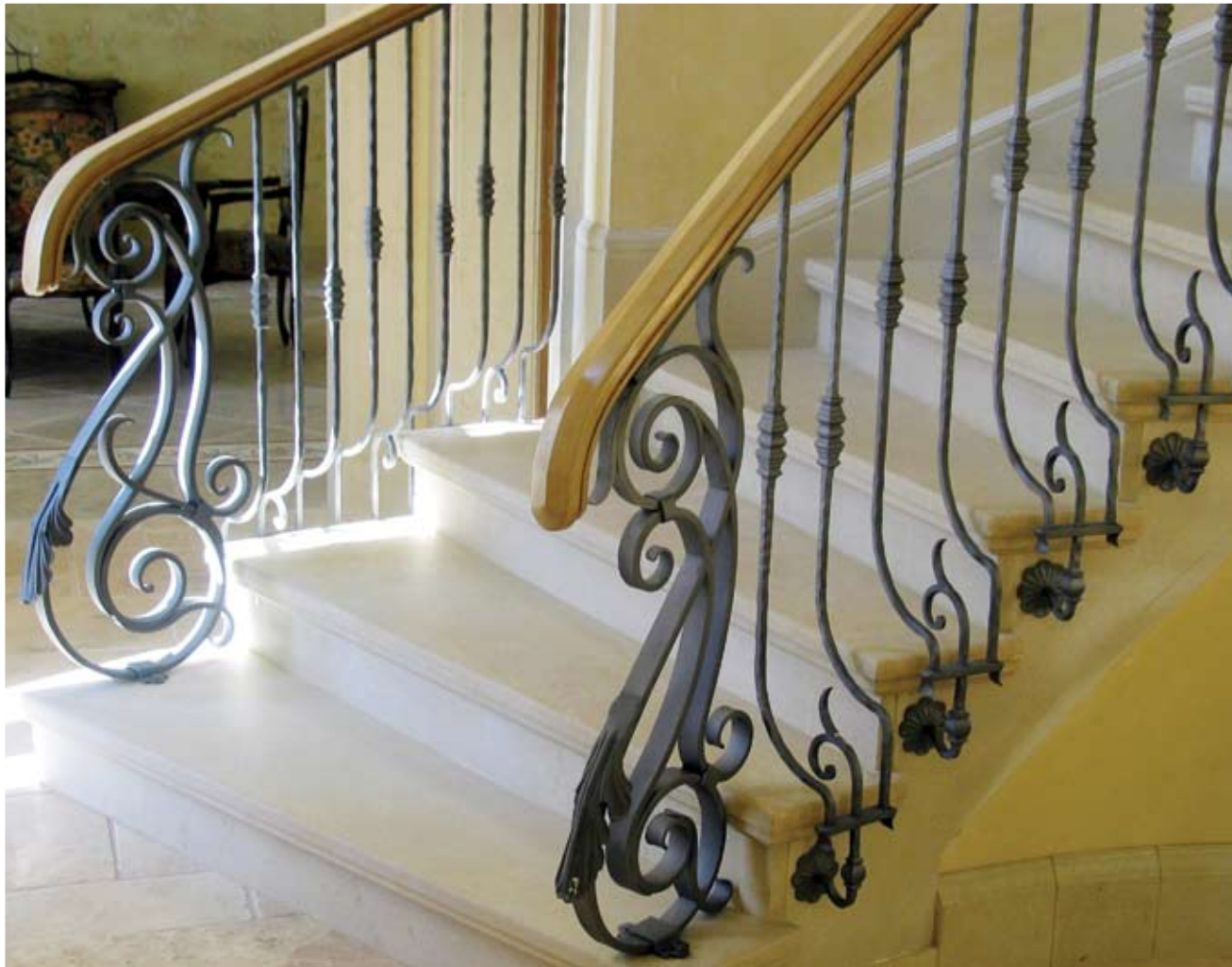
Forged silicon bronze railing and stanchions. Stanchion elements are all forged from 1x1 sq. bar. Design by Steve Austin. Inspiration source was Egyptian hieroglyphics. The ankh detail is a symbol of eternal life; the blade shape at bottom is a recurring form as are the "wings" in back of the ankh detail. Lead blacksmith: George Rousis.
