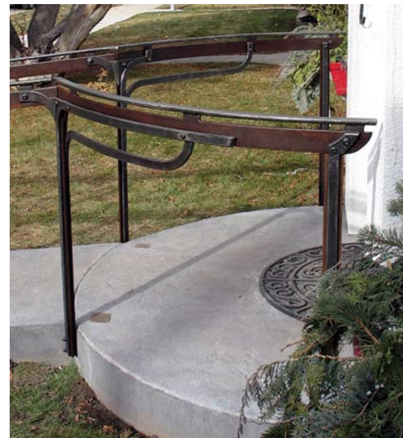
Entry railing detail.
