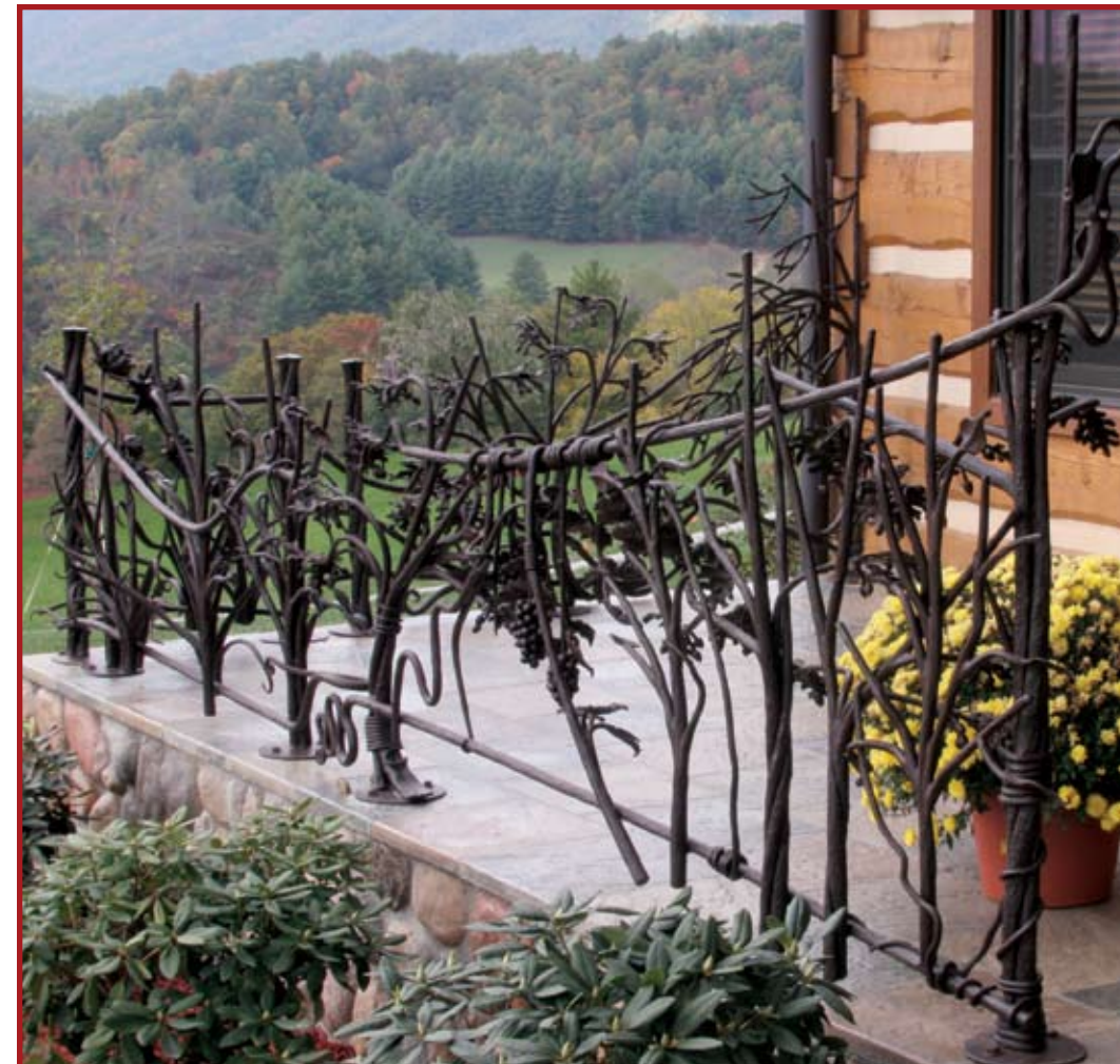
"Wildwoods" railing. Mild steel, forged and fabricated. Front and back views.
