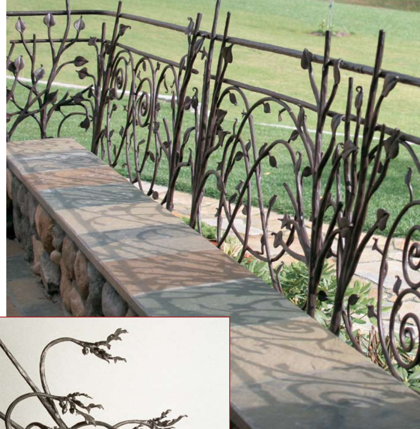
"Wildwoods" railing. Mild steel, forged and fabricated.
