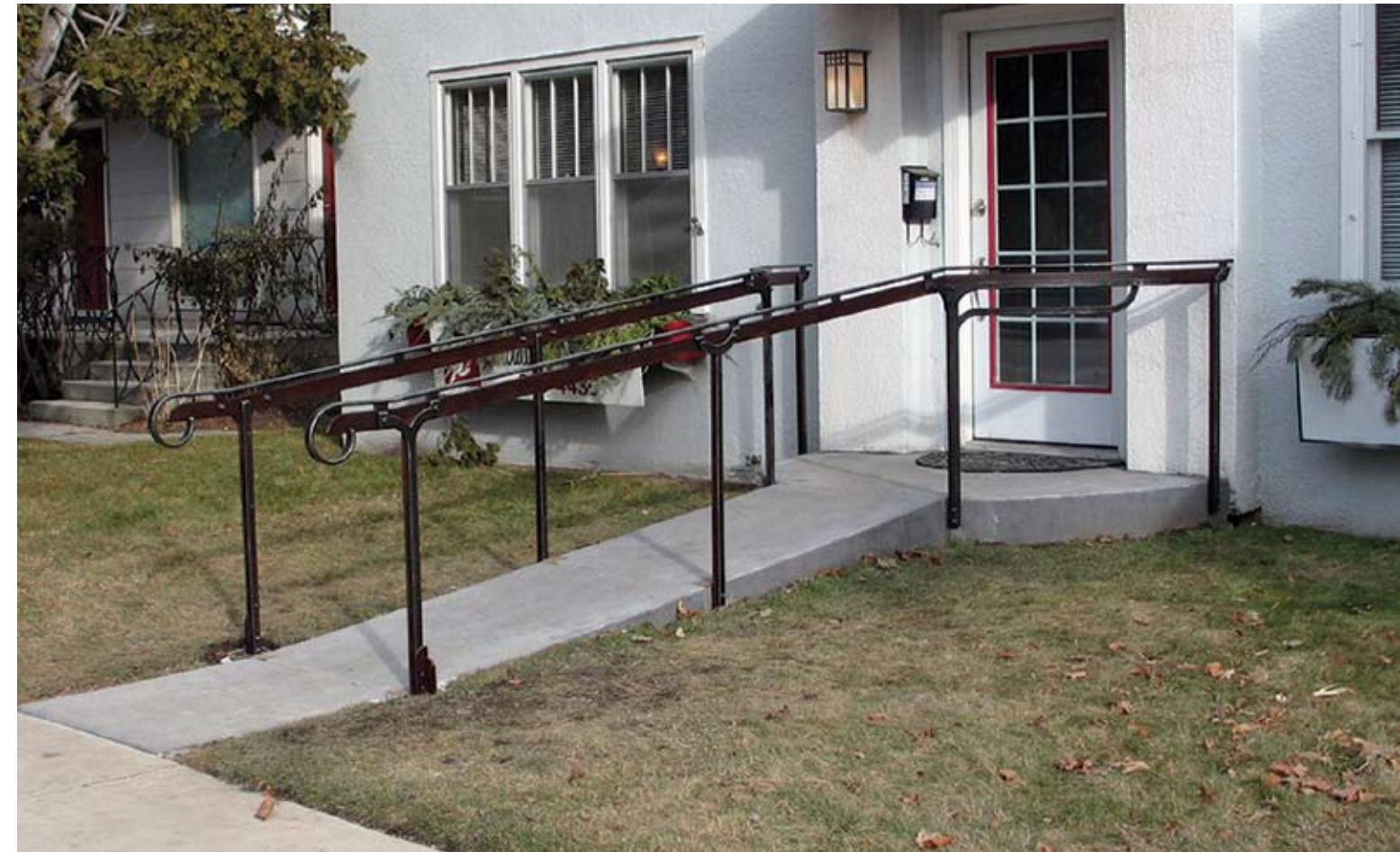
Exterior entry railing. At client's request, surface finish was to remain natural, and was treated with wax.
