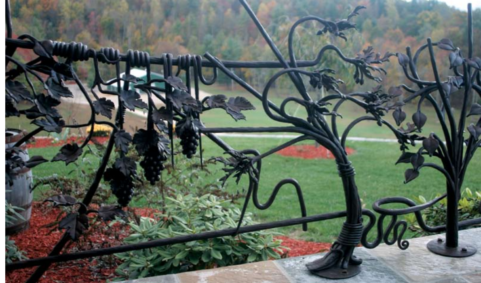
"Wildwoods" railing. Mild steel, forged and fabricated. Front and back views.
