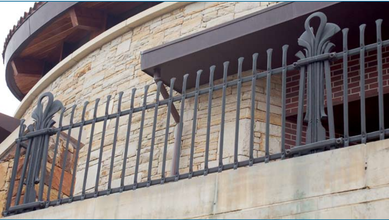
Forged silicon bronze railing and stanchions. Stanchion elements are all forged from 1x1 sq. bar. Design by Steve Austin. Inspiration source was Egyptian hieroglyphics. The ankh detail is a symbol of eternal life; the blade shape at bottom is a recurring form as are the "wings" in back of the ankh detail. Lead blacksmith: George Rousis.
