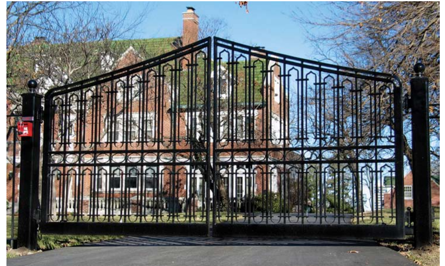
Motorized double entry drive gate. Forged and fabricated. Arch format is based on existing architectural detail of lintels above doorways and windows.
